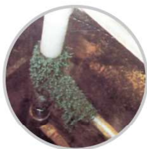
▲ When light penetrates in the tank : Moss and microorganism grow.
